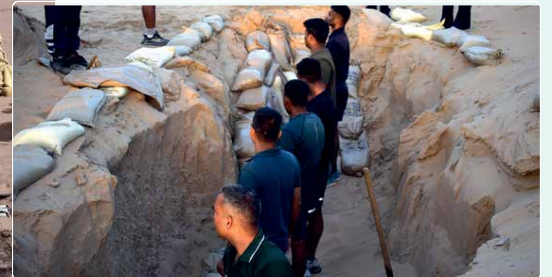
Unit personnel preparing trenches at Op location
